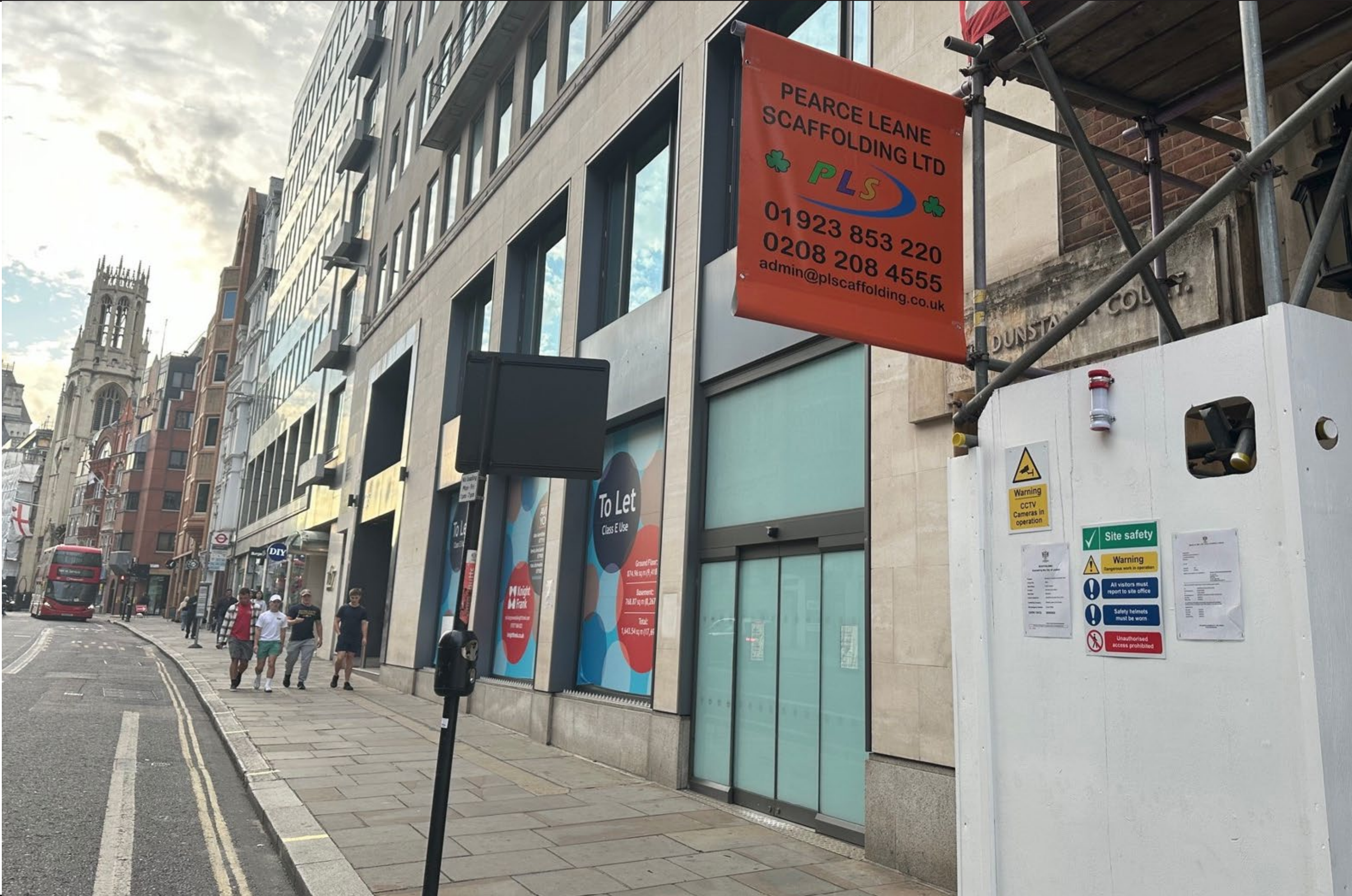
Existing Unit – Fleet Street View West
